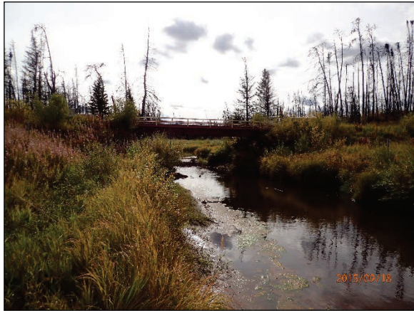
Hydrology Station S31: Hangingstone Creek at North Star Road, facing upstream
